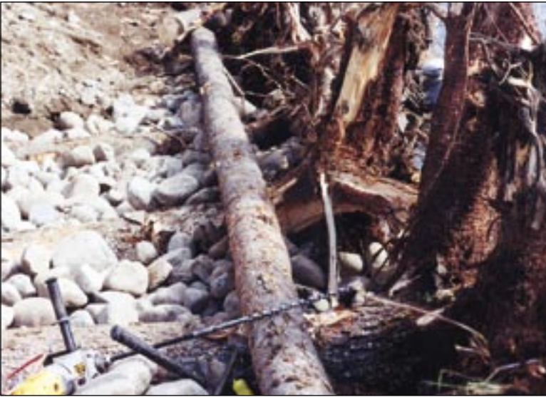
Root wad, rock layer with header log pinning, Pioneer Lodge
