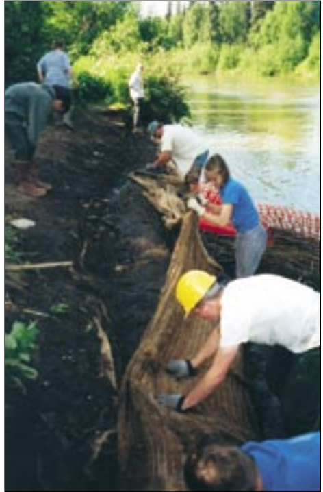
Installation of brush layering, Little Susitna River, Youth Restoration Corp.
