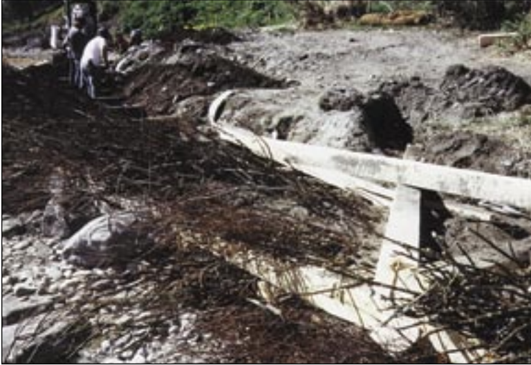
Vegetated cribbing project under construction. Note cross timbers. Kenai River.
