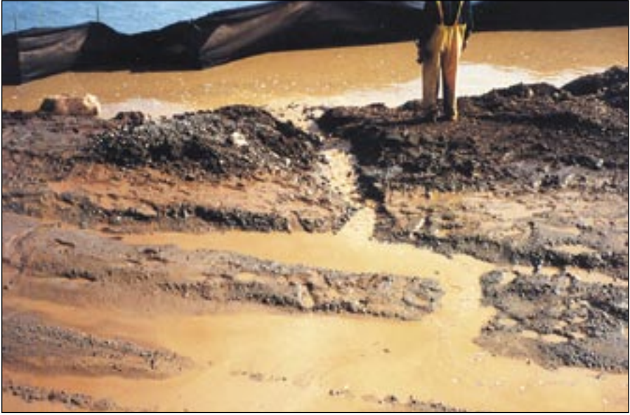
Centennial Park erosion control, Soldotna, Alaska
