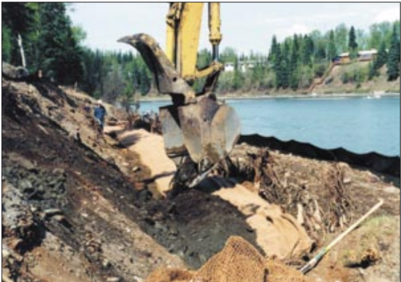
Rootwad and brush layering bank stabilization, Centennial Park, Kenai River
