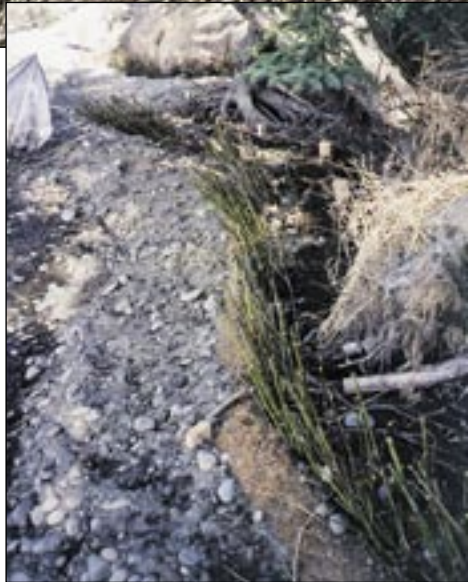
Live siltation protecting natural bank. Note partially buried coir log on riverside of live siltation.
