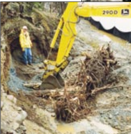
Root wad installation at Centennial Park, Kenai River
