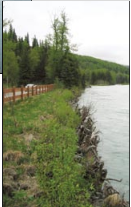
Jim's Landing brush layering/ root wad installation, Kenai River
