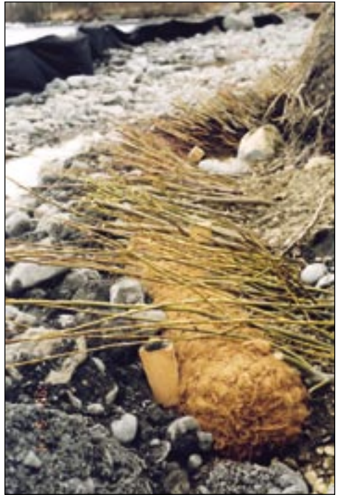
During installation with coir log toe protection, Eagle River
