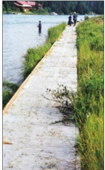
City of Soldotna Rotary Park angler walkway, Kenai River
