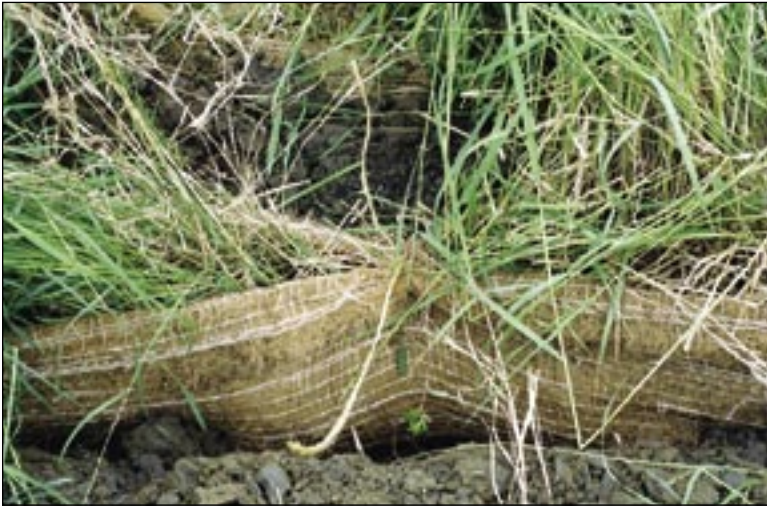
Detail, grass roll installation, mouth of Willow Creek
