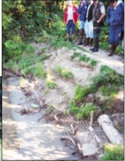
Little Susitna Recreation Site – Before Restoration
