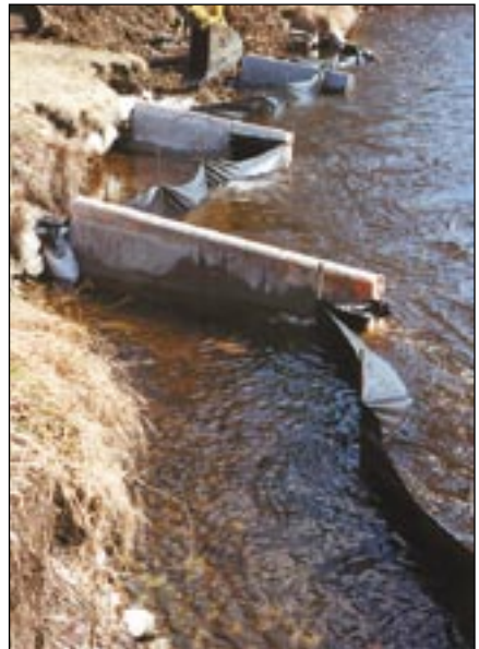
Jersey barriers and silt fence isolating the work area, Willow Creek
