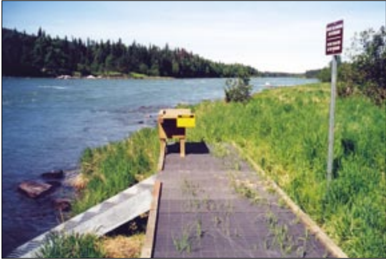
USFWS gratewalk with stairway to river for angler access, Kenai River
