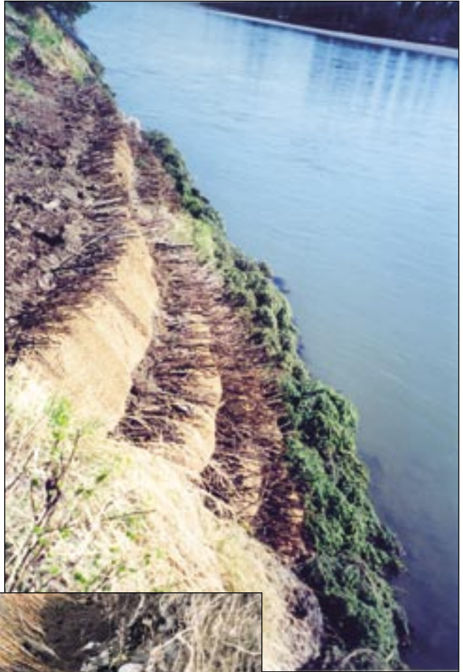
Brush layering and cabled spruce trees, Kenai River
