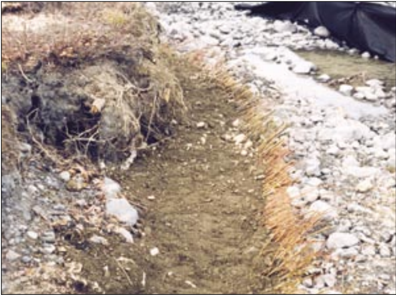
Live siltation during construction
