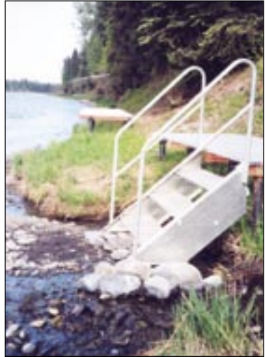
Gratewalk with stair to river bed for fishing access, Kenai River
