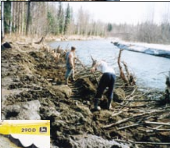
Installation of brush layering over root wads, Willow Creek
