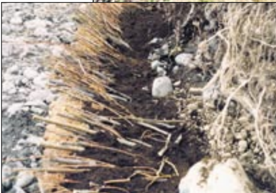
Detail, coir log toe protection
