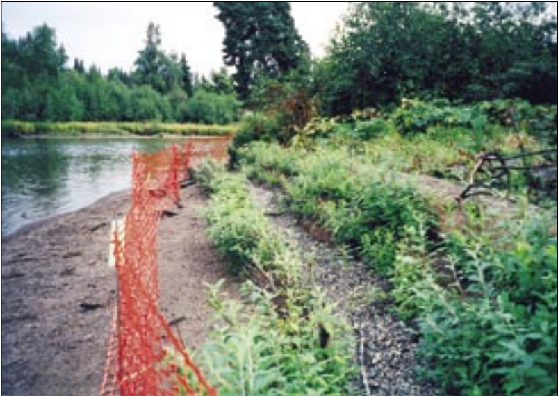
Little Susitna Recreation Site two months after brush layering and live siltation was installed
