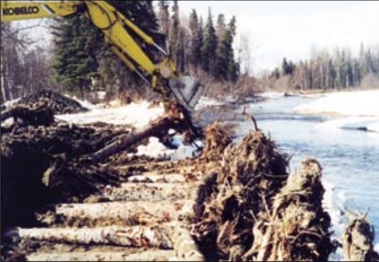
Root wad installation at Pioneer Lodge, Willow Creek
