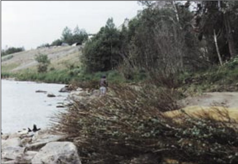
Vegetated cribbing three weeks after installation
