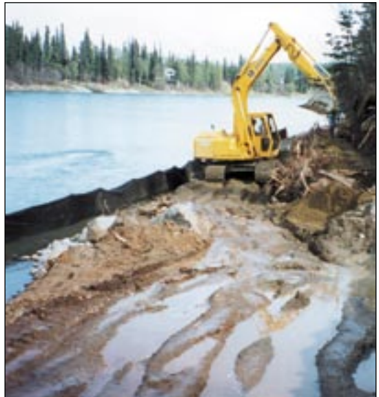
Excavator working at rivers edge with erosion control measures in place
