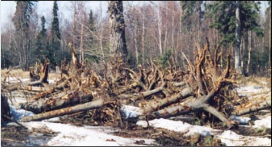
Harvested rootwads before installation
