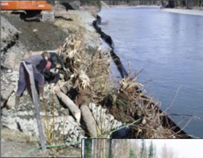
Pinning root wads with rebar, Jim's Landing, Kenai River
