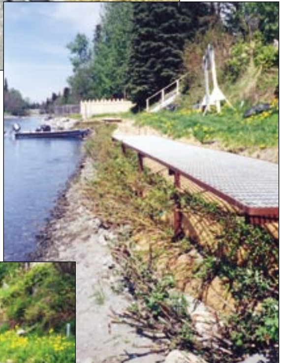
Live siltation and brush layering one month after construction, Kenai River
