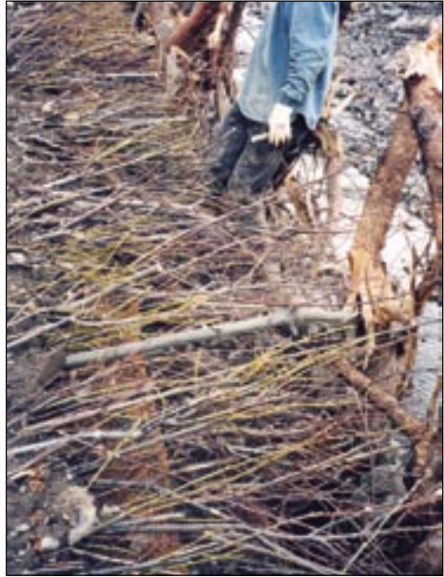
Brush layering installation prior to trimming, Centennial Park, Kenai River
