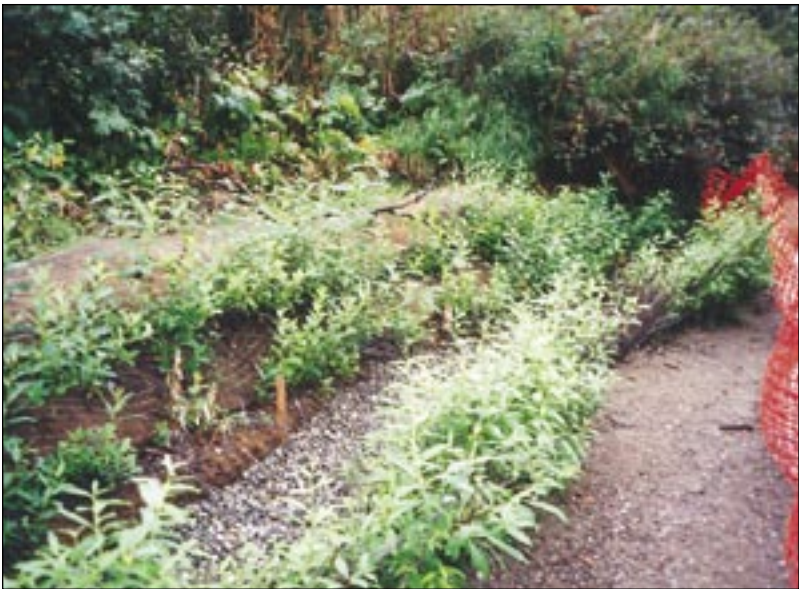
Live siltation and brush layering at the Little Susitna River
