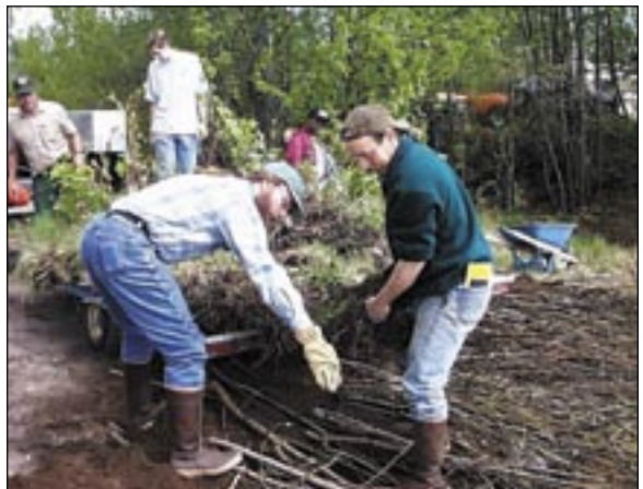
Placement of vegetative mat after harvesting
